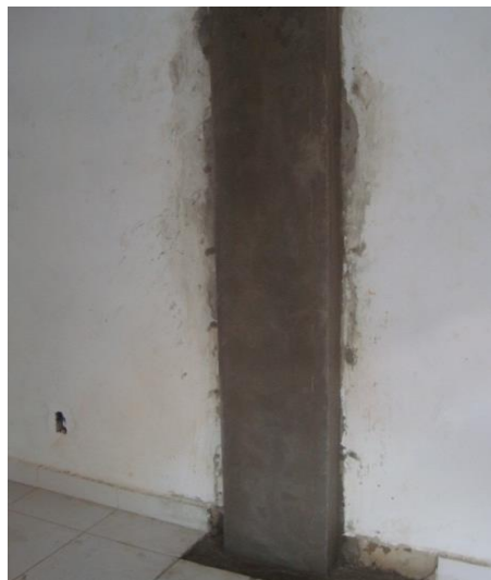
Figure 10. Final aspect of the strengthened columns.
