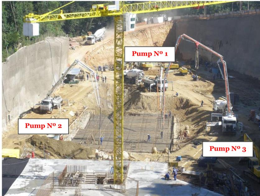
Figure 10. General view – Concrete pumps positioned.
