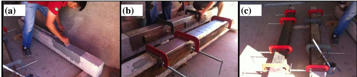
Figure 4. (a) Application of the epoxy adhesive to anchor the steel profiles; (b) Placement of the fasteners; (c) Final fastening system of the sheets.
