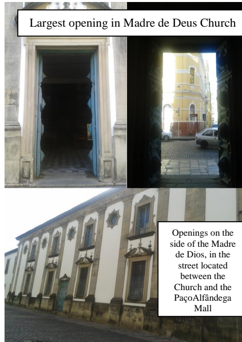
Figure 2. Openings for ventilation and exhaustivación of smoke of the Madre de Deus´ Church.
