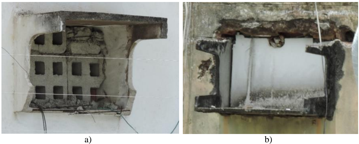
Figure 13. Partial break in open window model: a) absence of lower slab; b) absence of upper slab.
