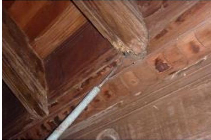
Figure 24. Investigation in wooden elements with graduated punch.
