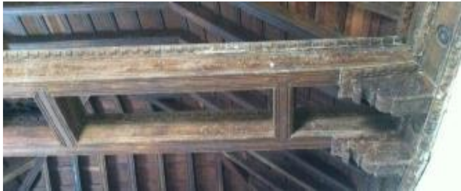
Figure 3. Tie rod beams on corbels.
