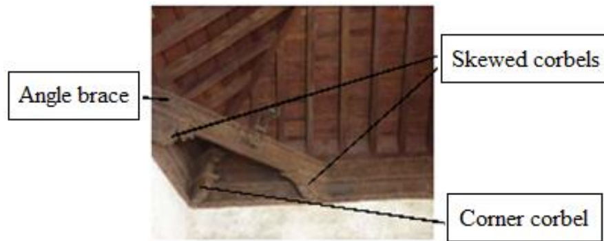
Figure 4. Angle brace, skewed corbels and corner corbel.
