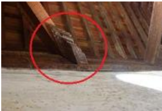
Figures 18 and 19. Dropping of skewed corbels (Sc7 and Sc8) under angle brace 4 (Ab4).
