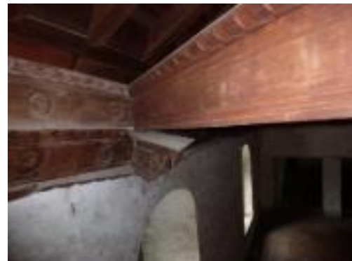
Figures 18 and 19. Dropping of skewed corbels (Sc7 and Sc8) under angle brace 4 (Ab4).
