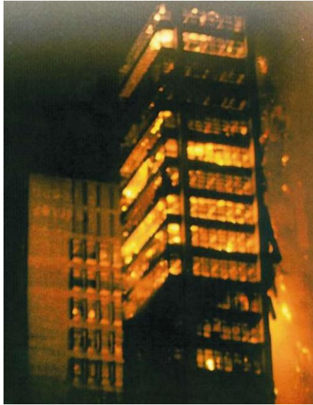
Figura 16. Building Sede II Remaining front
