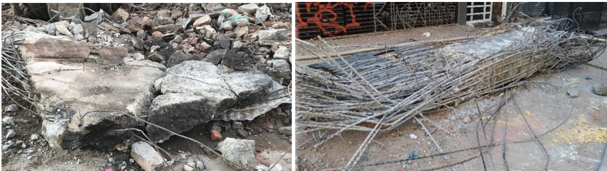
Figure 10. Excerpts cantilever slab and column collected from the debris for testing (source: Paulo Helene's personal collection)
