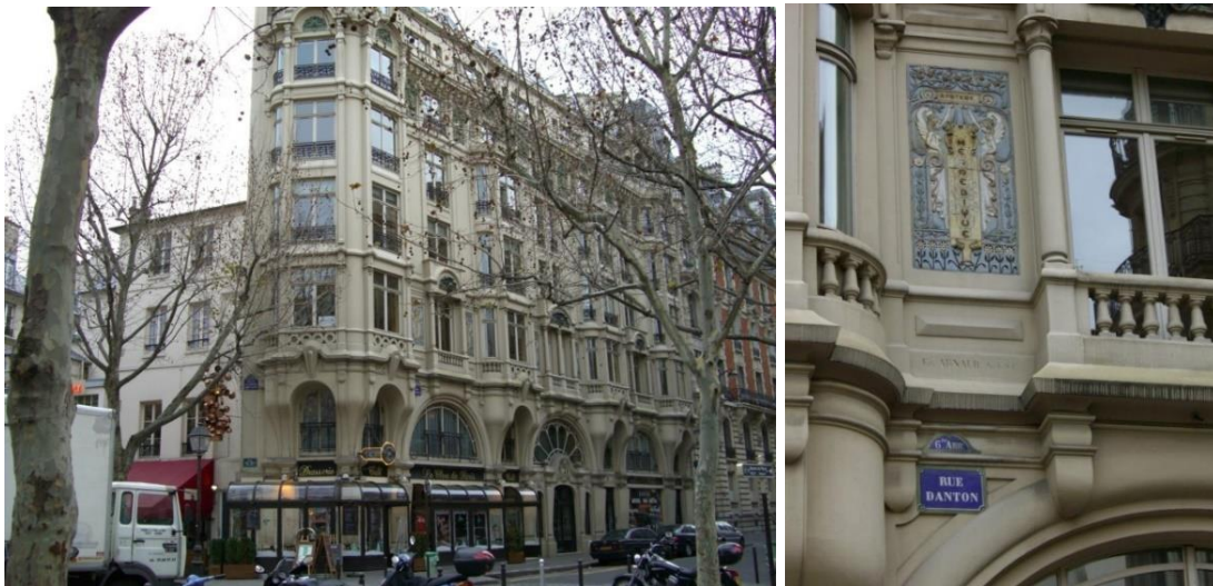
Figure 4. World's first building designed with the system Hennebique (119 years of good service to the society) (Source: Paulo Helene's personal collection).
