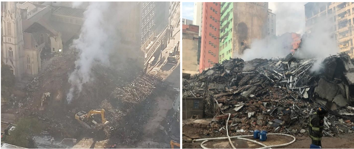
Figure 2. Wilton Paes de Almeida after its collapse (source: Paulo Helene's personal collection).
