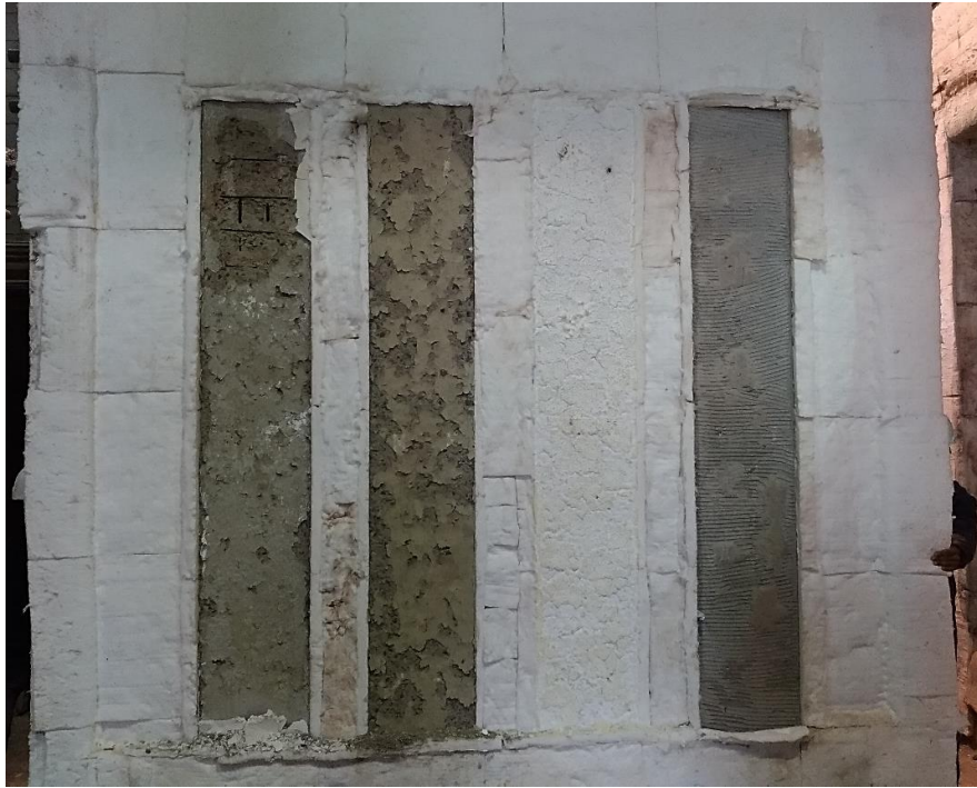
Figure 7. Detail of the elements and coatings condition after furnace opening (event 2): slow-set plaster coating, reference element, intumescent paint coating and cement-based mortar coating.
