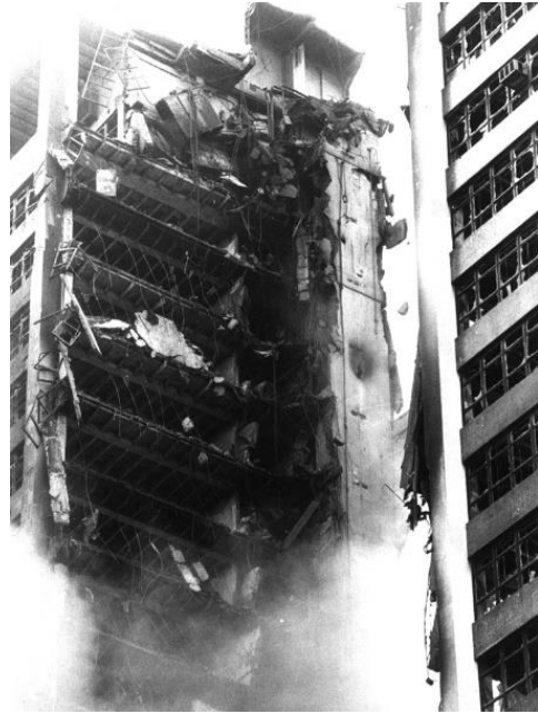
Figure 14. Detail of the Sede II building concrete structure collapse, showing the two remaining parts of the tower.
