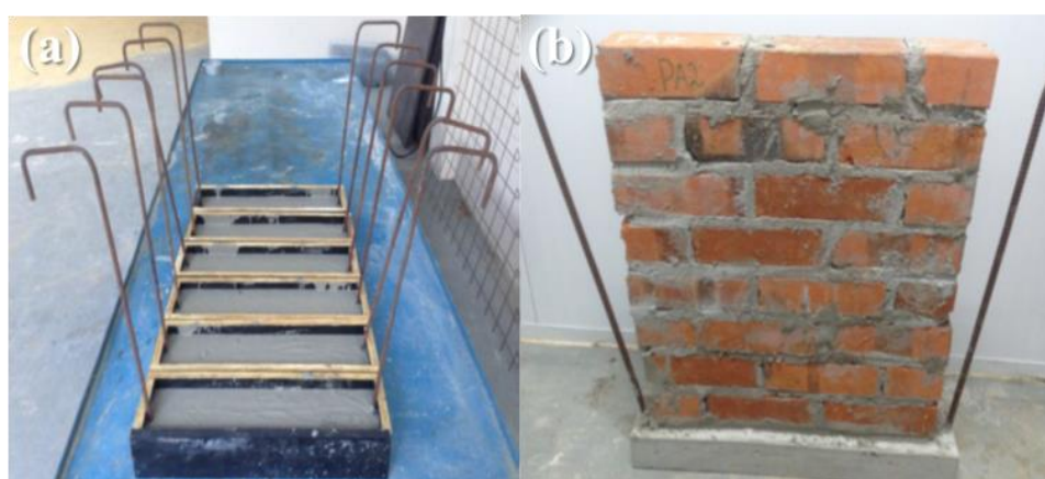
Figura 2. (a) Base de pared (b) Pared terminada
