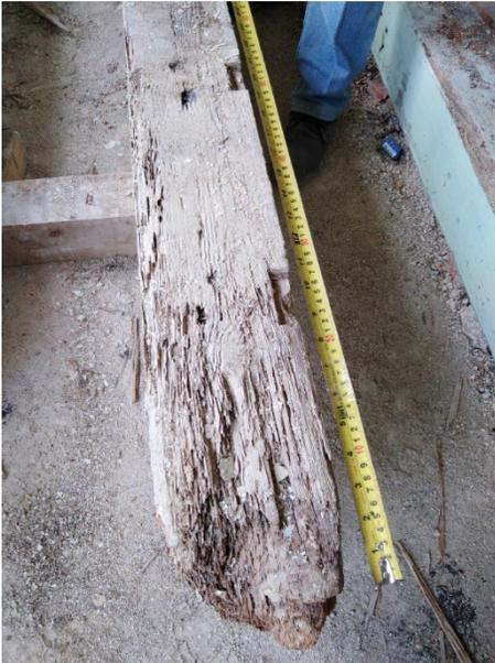
Figure 7. Measure of the affected beam section with Steel tape
