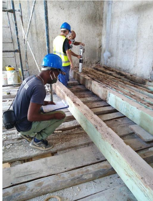
Figure 4. Inspection and visual classification of disassembled beams
