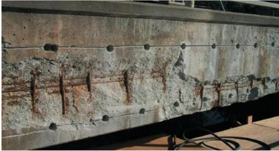
Figure 17. Discrete anodes on a bridge parapet.
