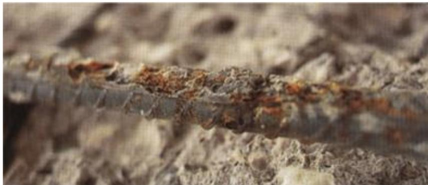
Figure 5. Typical pitting chloride induced corrosion.
